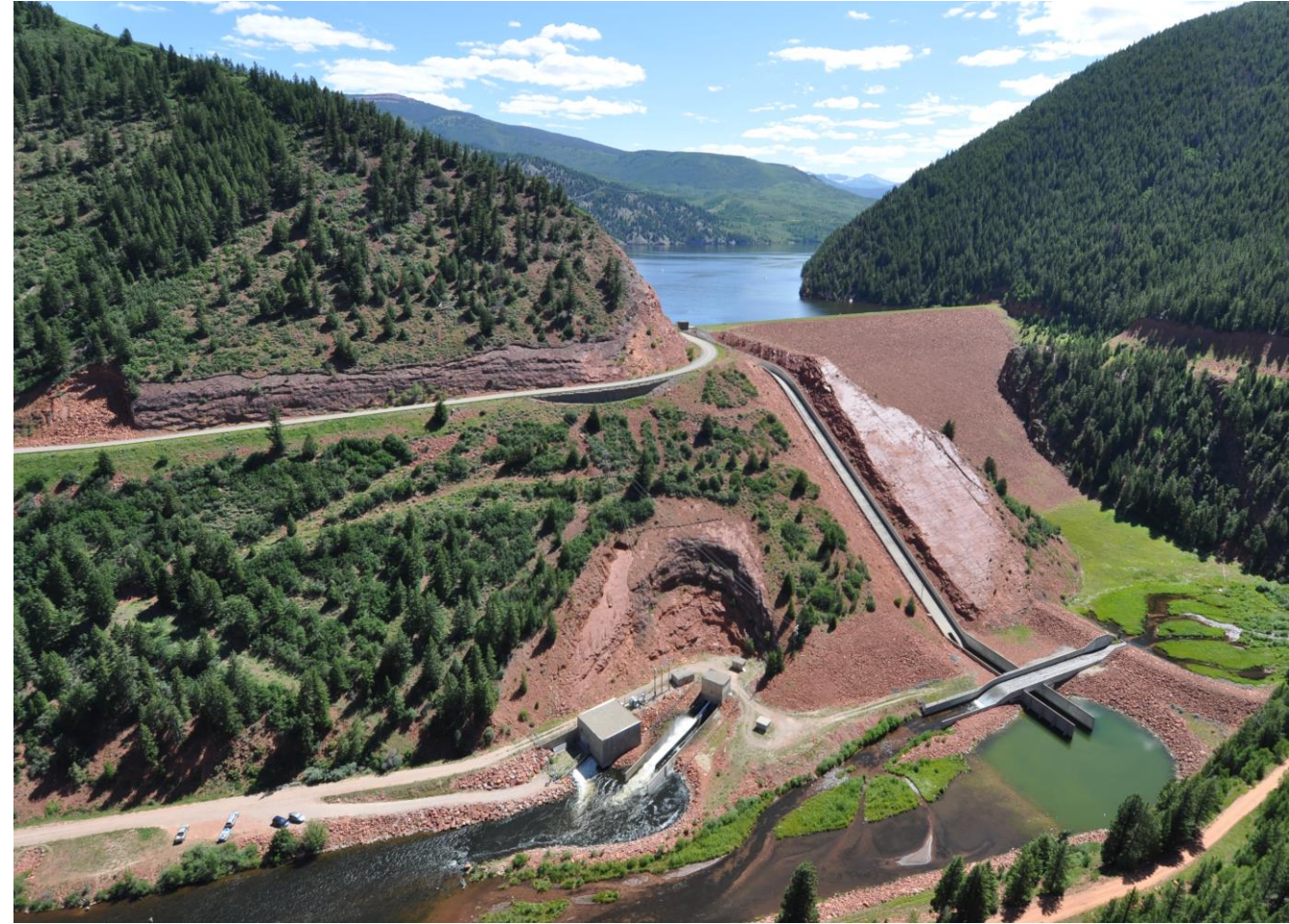
Ruedi Dam and Reservoir.
