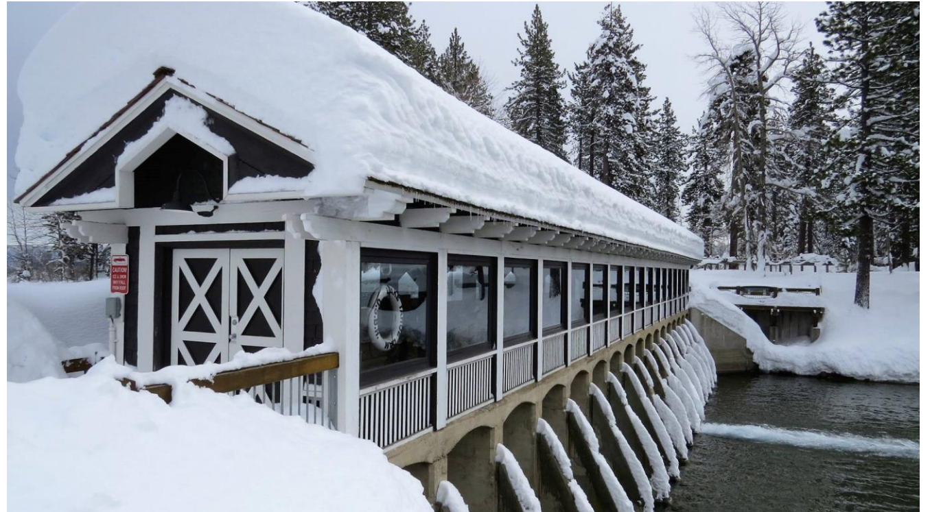
Lake Tahoe Dam winter 2017, photo credit Paul Larson
